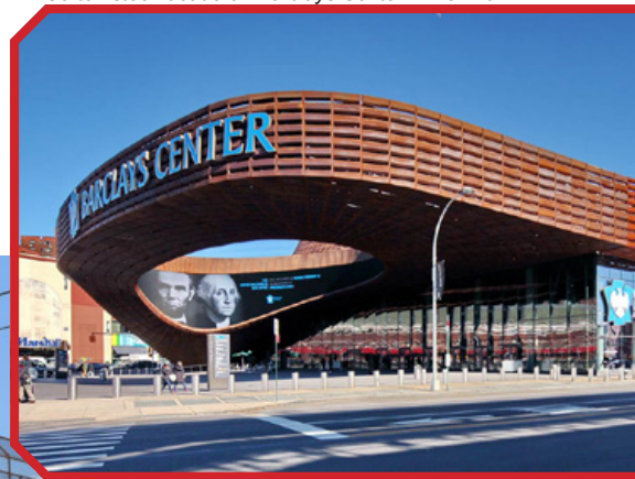
Corten steel facade on Barclays Center in New York.
