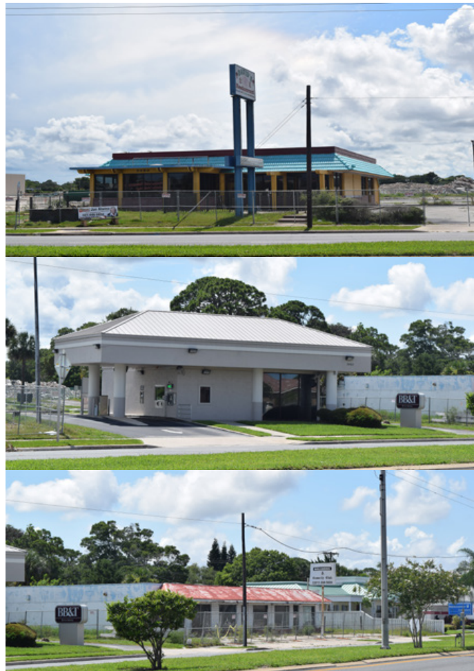
Above: Outparcel B of Titus Landing, before demolition began.
