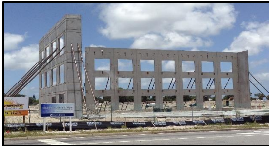
New PMC Building Under Construction at Titus Landing
