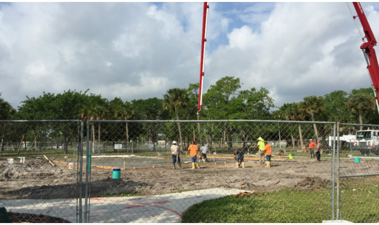
Foundation pouring at the splash pad.
