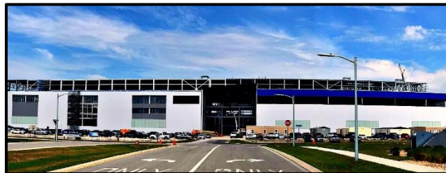
Blue Origin Facility, Under Construction
