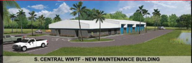
S. CENTRAL WWTF - NEW MAINTENANCE BUILDING
