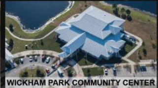
WICKHAM PARK COMMUNITY CENTER
