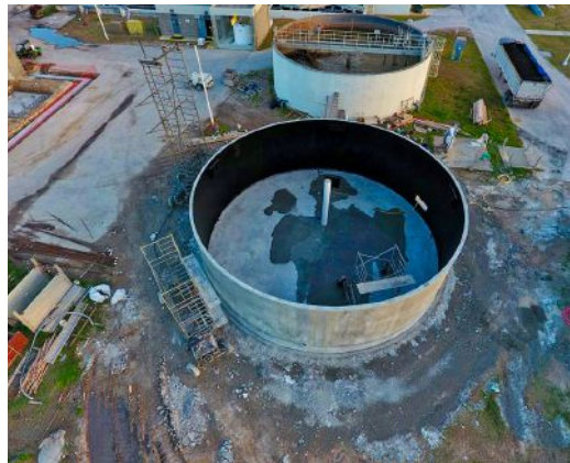
Expansion at the South Central Regional Wastewater Treatment Facility will help the County meet growing demand on the infrastructure.
