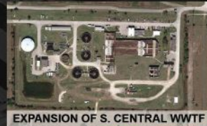
EXPANSION OF S. CENTRAL WWTF
