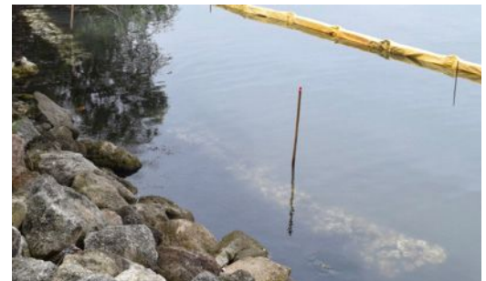
View of newly installed native vegetation at the Eastminster shoreline. Rock revetment is more effective when partnered with native coastal marsh plants and an oyster reef breakwater. The plants and oyster shells provide habitat and food for marine life such as red drum, flounder, blue crab and shorebirds and help slow erosion of the rip-rap barrier.
