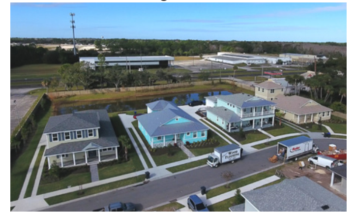
Several homes have been completed and more homes are under construction at the 22-lot subdivision located on Riveredge Drive.
