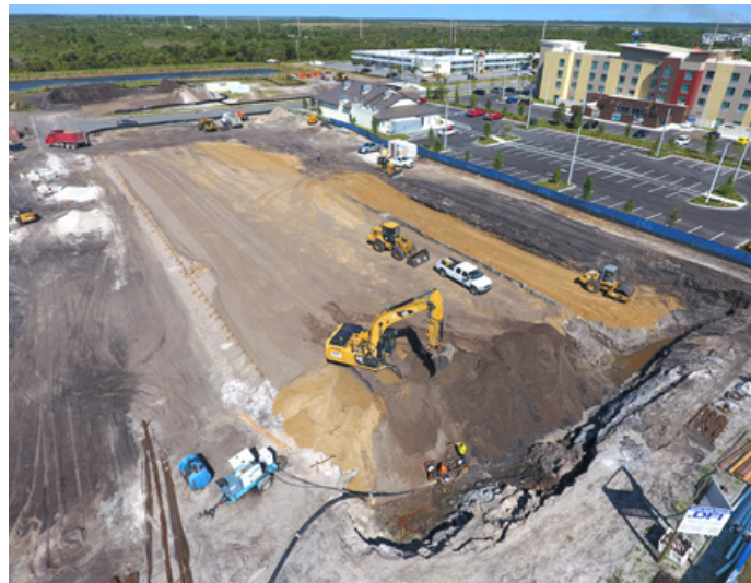
Construction has begun on a 124-unity, 4-story hotel located at the southern terminus of Helen Hauser Boulevard adjacent to the new Durango's restaurant.
