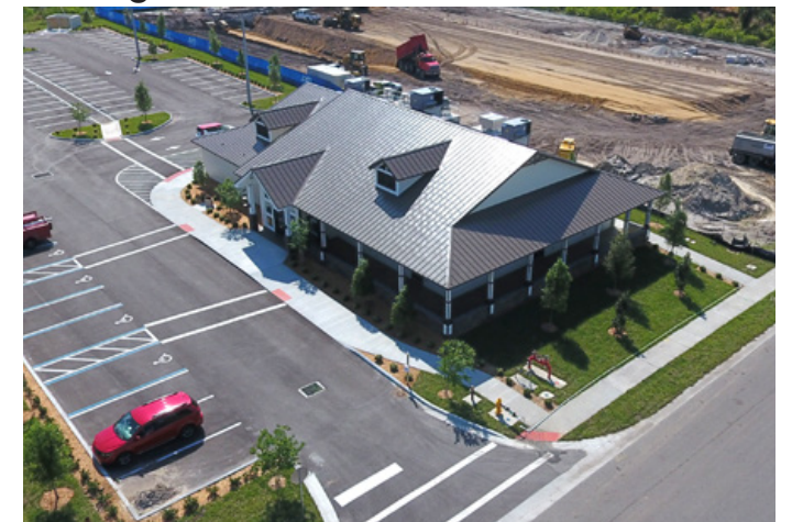
Construction is nearing completion for a 6,600-square-foot restaurant located along Helen Hauser Boulevard, south of S.R. 50.
