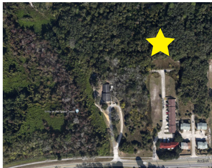
Site plans are under review for an 18,000-square-foot children's daycare center located north of South Street and west of S. Park Avenue.
