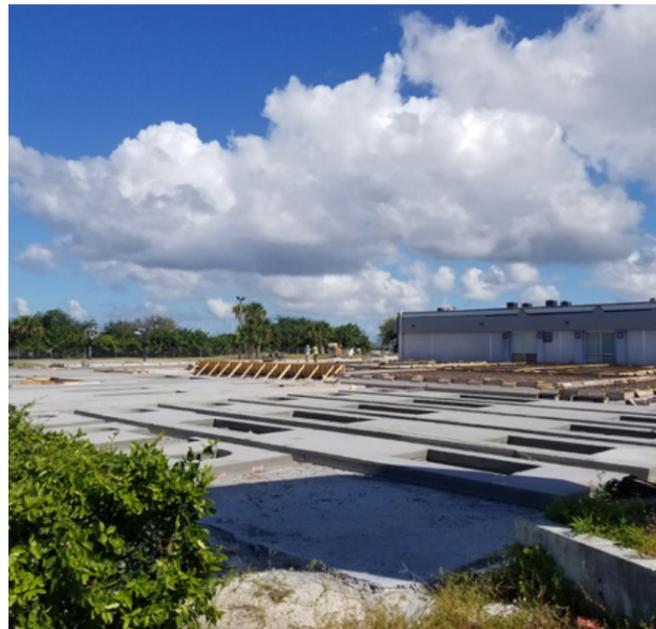
Construction is underway on a 4,900-square-foot addition to the St. Stephen's Christian Retreat Center on US 1 south of SR 50. The new building will be used for assembly and conference functions. The photo above shows the concrete tilt walls recently formed and poured. These tilt walls will soon be erected by cranes and secured to form the new building.
